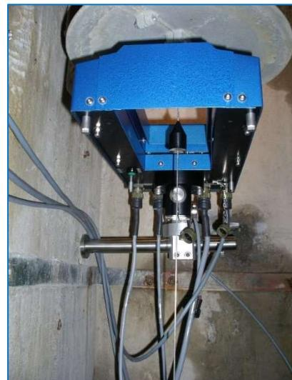
After main construction work was completed, a set of direct and inverted pendulums, partially equipped with manual operated and partially with automatic pendulum measuring devices not originating from Huggenberger AG, has been installed.
